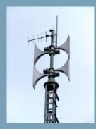
One of the most generally usable early warning technology is to use a public alarm system formed by electronic sirens installed in the endangered areas (e.g. the settlements around a factory or along the seaside, or even in the factories themselves).
